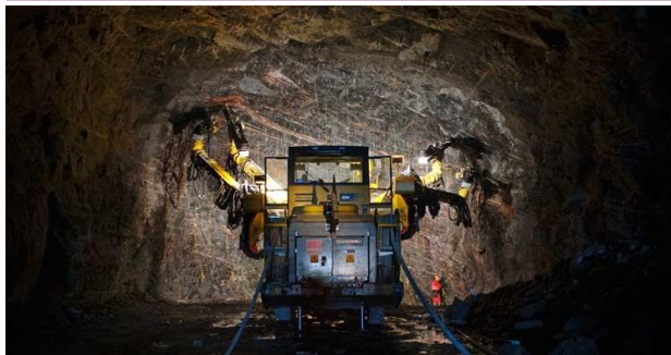
Underground civil engineering
