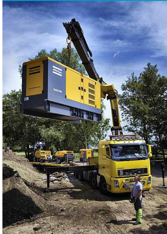
Power On-site generators
