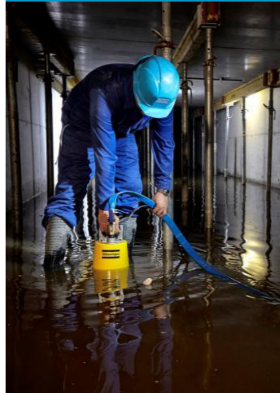
Water On-site pumps
