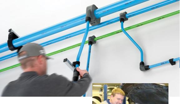
Expressway's AIRnet system provides air for pneumatic tools in the service department and in the lube center. Oil-fired heaters are used in the service areas and the AIRnet system supports those systems as well.
